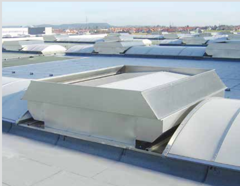
Section of Apollo ATI in closed position
