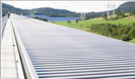
Colt's Labyrinth industrial ventilator achieves high capacity, weatherproof ventilation using aerodynamically shaped louvres.
