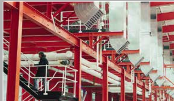
Colt's inflow unit warms, re-circulates and filters heating air.
