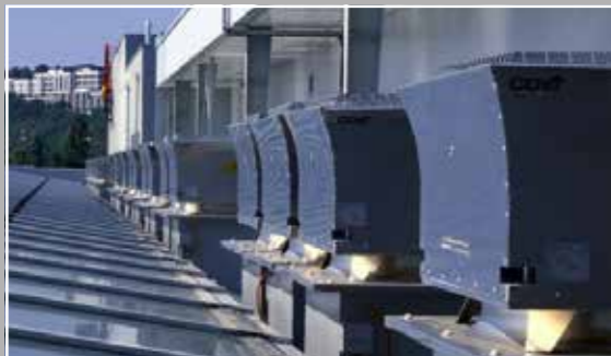
Colt's Liberator powered ventilator can be roof or wall-mounted.
