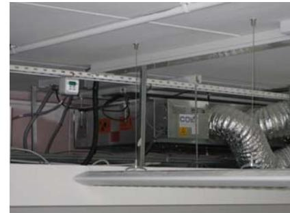
*Caloris WRF unit installed within purpose built bulkheads*
