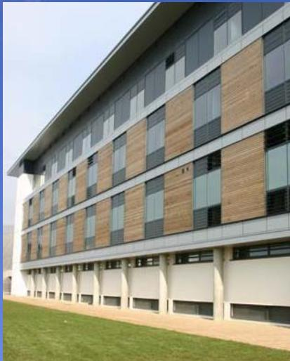
*Coltlite is a natural glazed ventilator for installation into the facade which can provide both day to day and smoke ventilation. Its form and function make it particularly suited to educational buildings where good U values and low air leakage are required.*
