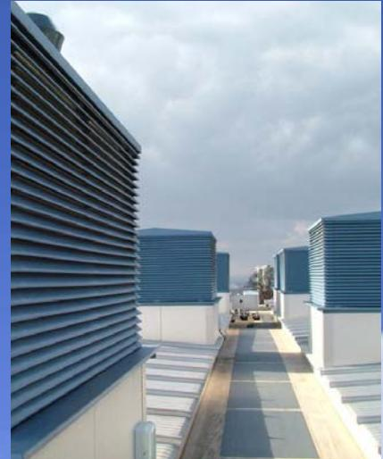
*Colt Turret units are available in a wide range of standard sizes in Single bank or Double bank configurations. Colt Turrets are available in a complete range of finishes and materials from standard mill finish and polyester powder paint finish to anodised and stainless steel.*
