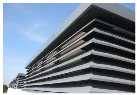
Roof top double bank louvre turrets with internal controllable dampers to regulate the flow of air and eliminate rain entry.
