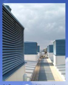
Colt Turret units are available in a wide range of standard sizes in Single bank or Double bank configurations. Colt Turrets are available in a complete range of finishes and materials from standard mill finish and polyester powder paint finish to anodised and stainless steel.
