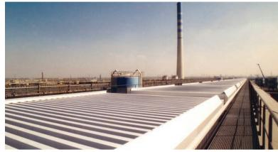
In 1980 Colt was required to replace existing mechanical HVAC equipment at Trimet aluminium in Essen, Germany in response to changing needs, and supplied a scheme of natural/gravity ventilation. This scheme consisted of a Labyrinth Ventilation system and wall louvres. Now, after more than 30 years of operation the system is still in a very good condition and shows no sign of destructive corrosion.
